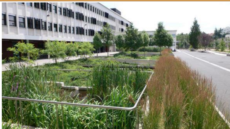
A rain garden can take the form of a series of planted basins, as seen here in the redesigned courtyard of the Lycée Saint Exupéry, Lyon, France. Source: Cerema
