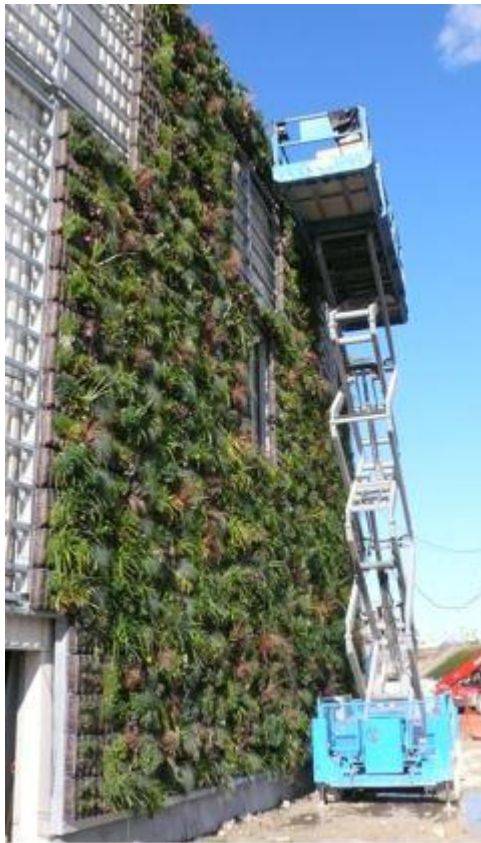
Figures: implementation of the elements of a green wall under construction at the Shopping Mall "Les Sentiers" in Claye-Souilly; and Green façade with climbing plant.
