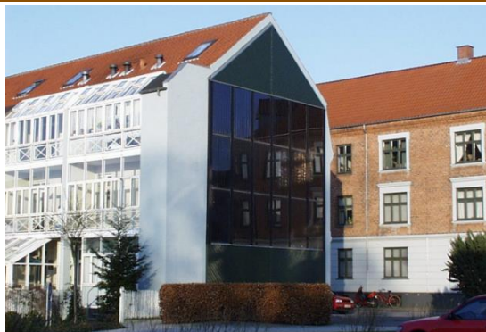
Building integrated solar thermal – flat plate collectors [1]
