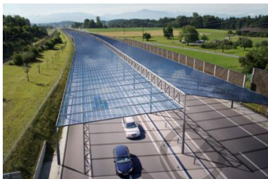
Photovoltaics in roads [4]
