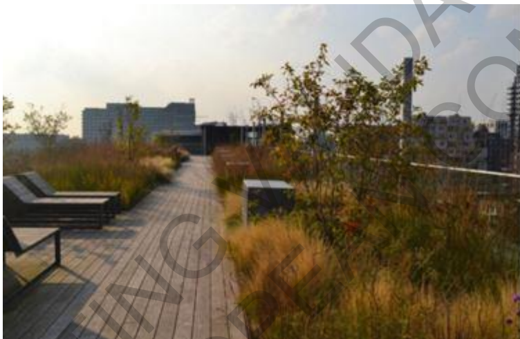
Blue-Green Roof in Amsterdam (source: RESILIO Project; https://resilio.amsterdam/en/ )
