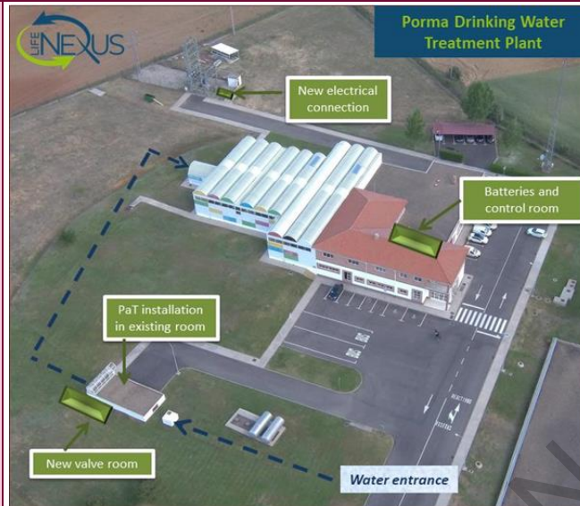
Indicators for the installation in Porma DWTP
