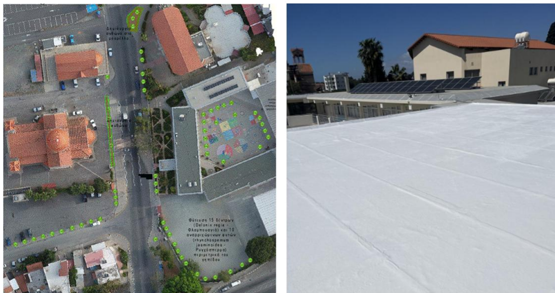
Figure 13 : Cool Roof and Greening Interventions in Limassol
