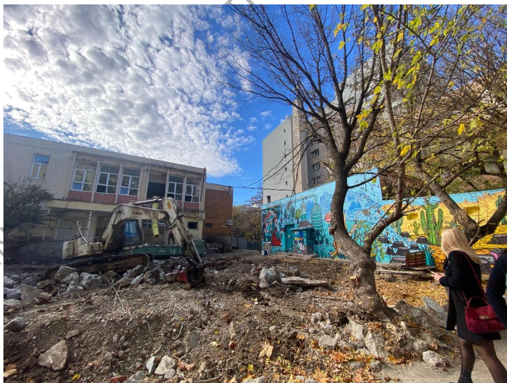
Figure 6 - Visiting the UrbanWise pilot site at Campus Verde, Bucharest — where concrete surfaces are being removed to restore the soil's natural capacity, making way for green, permeable spaces that reduce flood risk, and lower temperatures during heatwaves.
